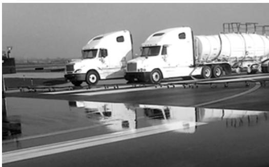
The photo above was taken shortly after the pavement had been washed during the runway grooving. Note the sharp dividing line between the grooved portion, where water rapidly drained off, and the ungrooved portion, showing the reflection of the trucks in the standing water.
