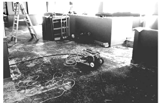
Dining room renovation in progress
