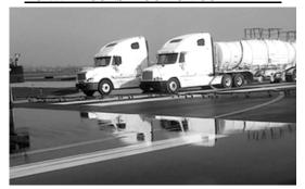
The photo above was taken shortly after the pavement had been washed during the runway grooving. Note the sharp dividing line between the grooved portion, where water rapidly drained off, and the ungrooved portion, showing the reflection of the trucks in the standing water.
